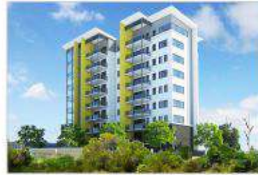
KINGDOM TOWER Thokkottu, Mangalore.
